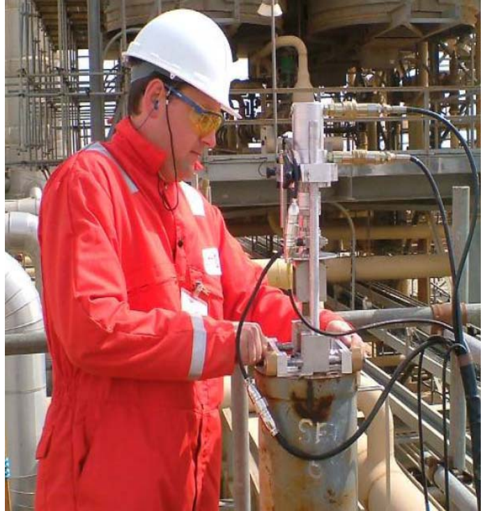
On site testing of safety relief valve 'In Situ'
