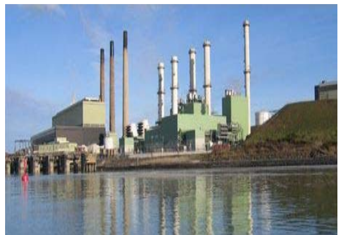
Ballylumford's 600MW Power Station
