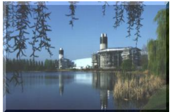
Barking's 1000 MW Power Station
